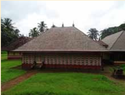
Shrines inside the temple premises
