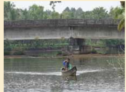
New bridge over Kavvayi river
