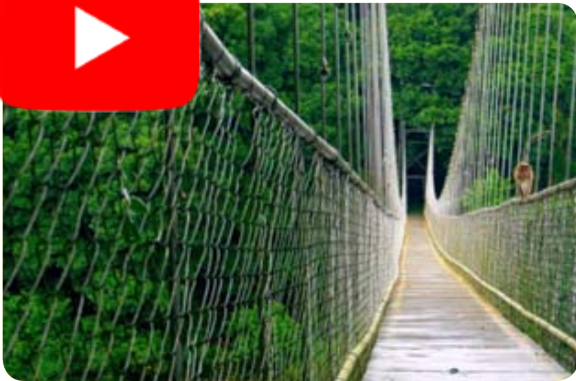
Hanging Bridge at Nilambur
