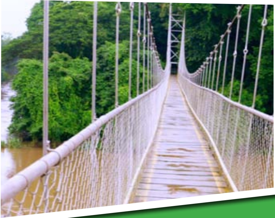
The hanging bridge at Nilambur
